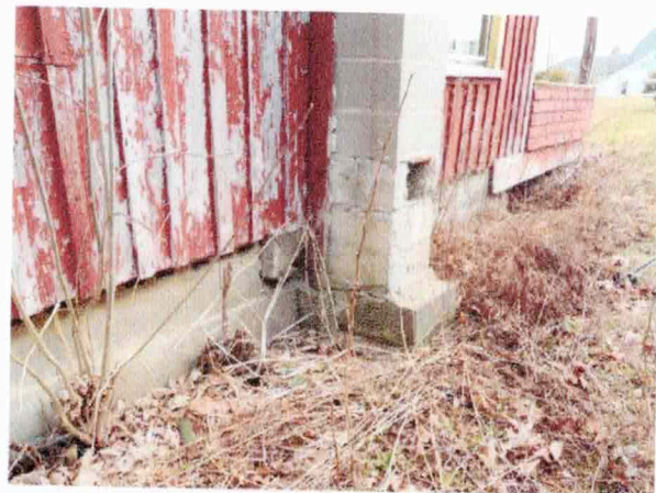
12) Exterior – West CMU chimney has significant cracks and spalling at the base
