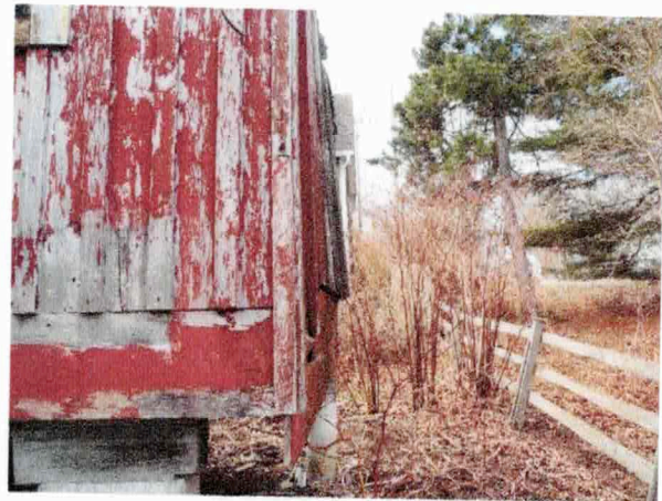
10) Exterior – North addition has significant bulges in the exterior walls, suggesting structural failure in the wood framed walls
