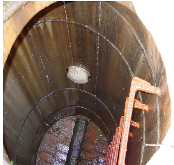
Before repair photo of MH 2025
