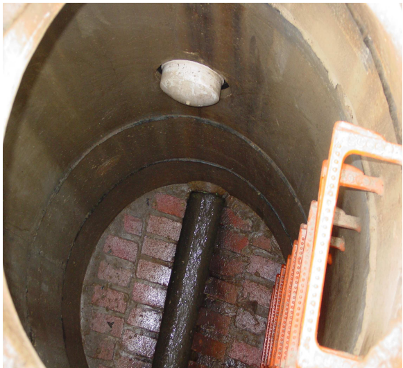
After repair photo of MH 2025 Chlorination/Dechlorination System
